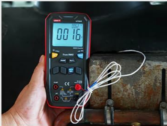
Refrigeration system inspection
