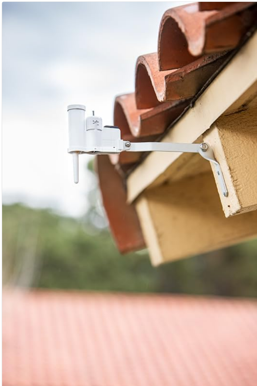
Figure 4: Hunter Wireless Mini-Clik Sensor mounted on an eave. This image demonstrates a typical installation location for the sensor unit, ensuring exposure to rainfall.
