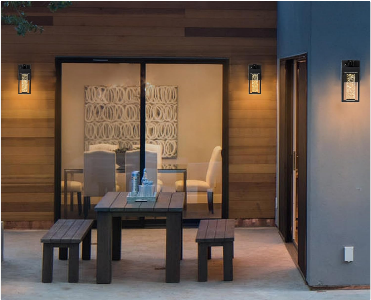
Figure 7: Versatile use of GFCI outlets for various outdoor equipment.
