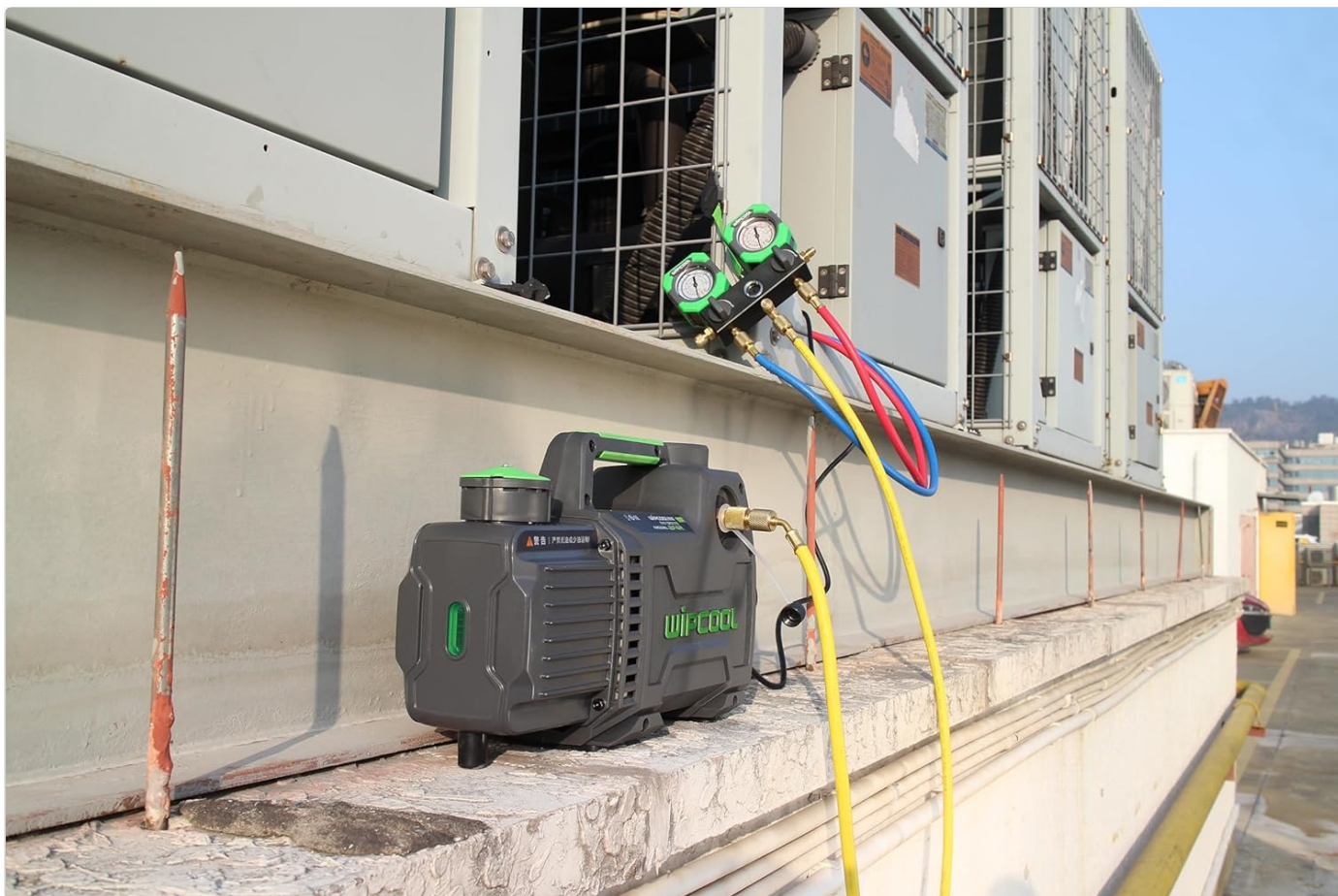
Figure 3: The Wipcool 2F3R vacuum pump in operation, connected to an HVAC system for evacuation. This image demonstrates a typical setup during use.
