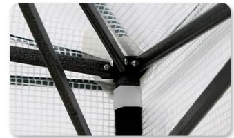
Double layer reinforcement at corners and peak
