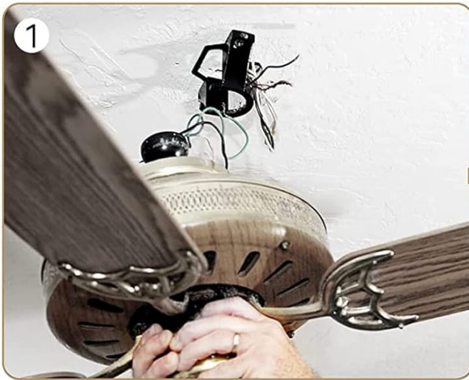
1 Disconnect the ceiling fan wiring
