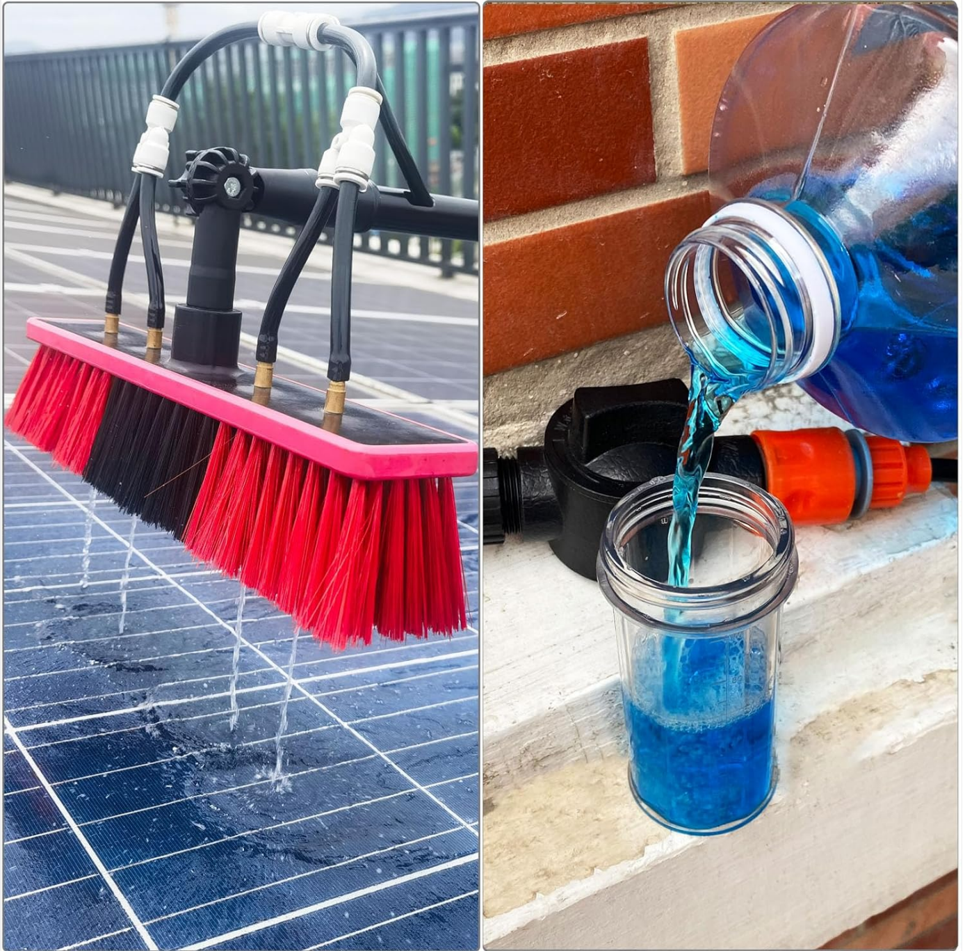
Image: The water-fed brush cleaning a solar panel, showing water flowing through the bristles. Another image shows a person pouring cleaning solution into the soap dispenser, demonstrating how to prepare for soapy water cleaning.
