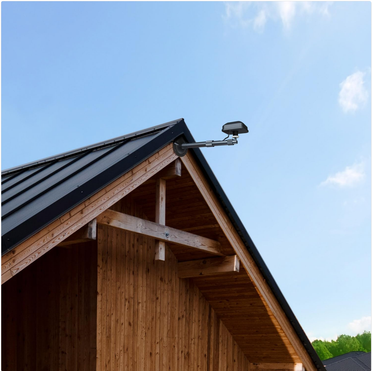
Figure 3: Example of GNSS antenna installed on a rooftop.
