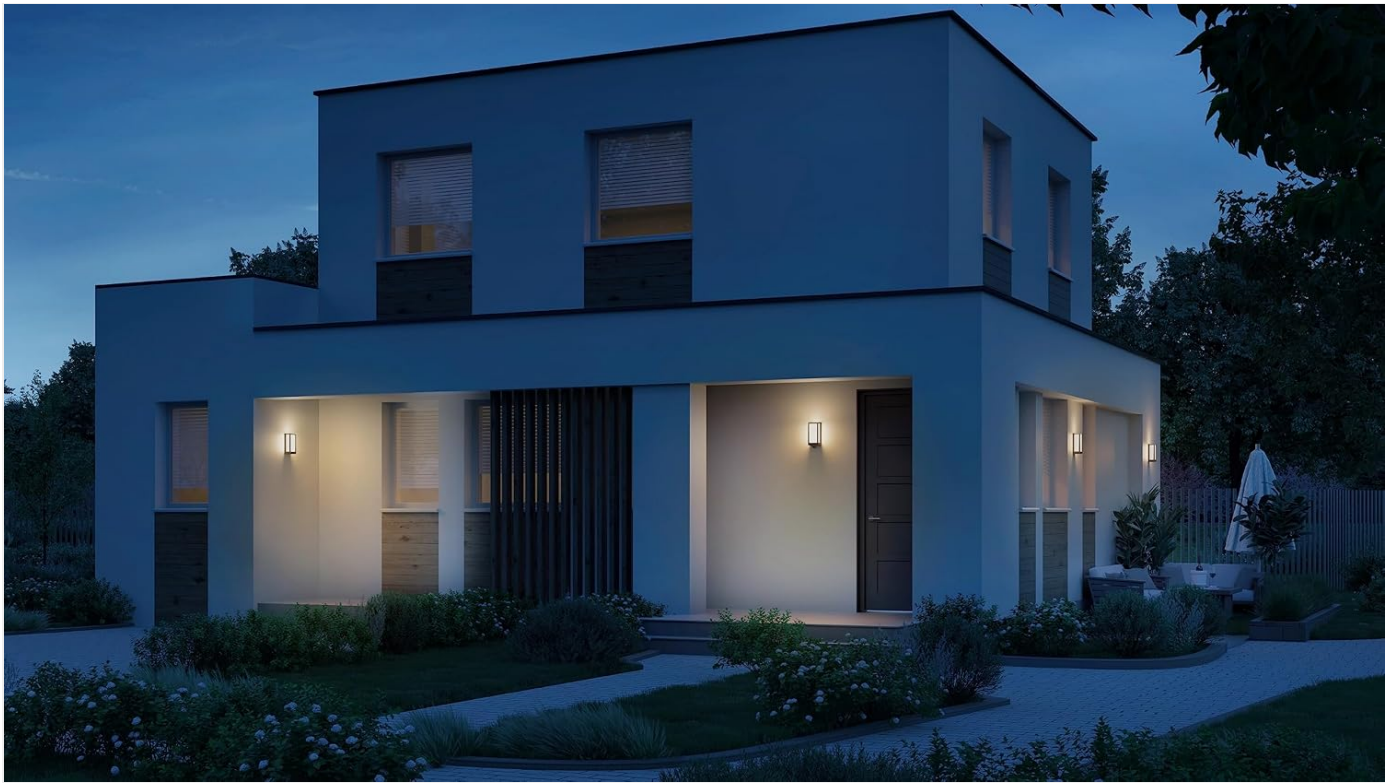
Image: An exterior view of a modern house featuring multiple Steinel L 42 C LED Outdoor Lights illuminating the facade, entrance, and patio areas.
