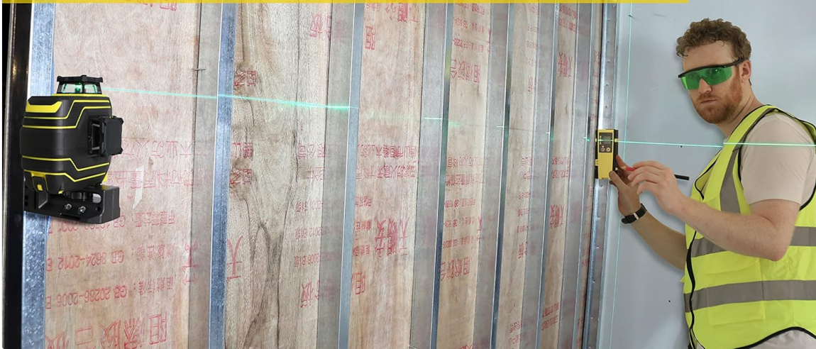
Figure 6.2: Using the Laser Level with a Detector in Pulse Mode.
