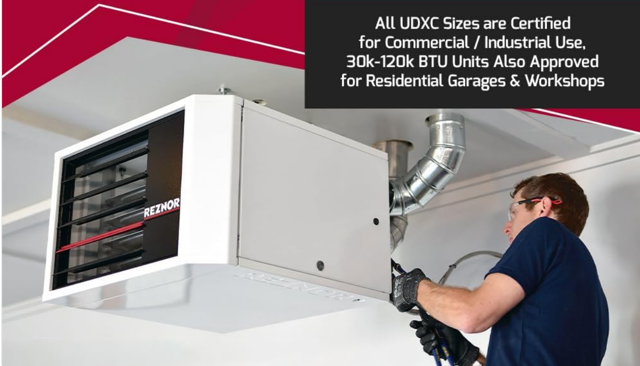
Figure 3: Installation of the Reznor UDXC-150 Heater. A worker is shown connecting ductwork to a ceiling-mounted heater. The text emphasizes the unit's suitability for commercial/industrial spaces, corrosion-resistant materials, and quiet, efficient heating.
