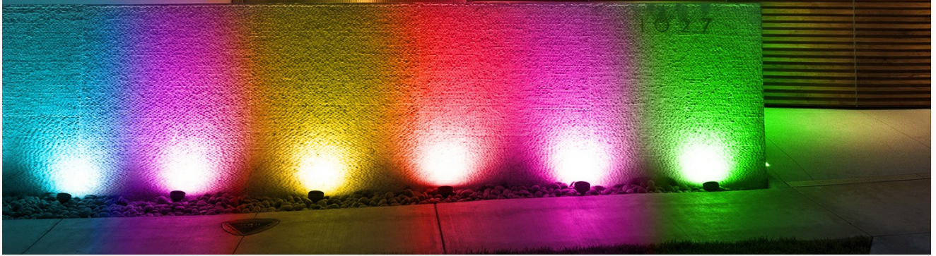
Figure 5.2: Individual control of each spotlight, allowing for diverse color arrangements.
