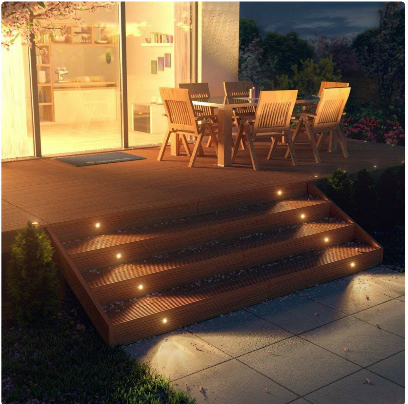
Image 5.2: A nighttime view of SMY Lighting recessed deck lights installed on outdoor wooden stairs, providing clear and safe illumination for pathways.
