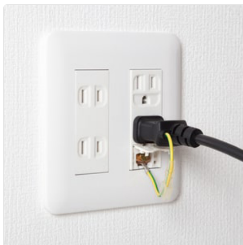
Image: A 2-pin power plug with a visible ground terminal (green and yellow wire) properly connected to a wall outlet, emphasizing the importance of grounding.
