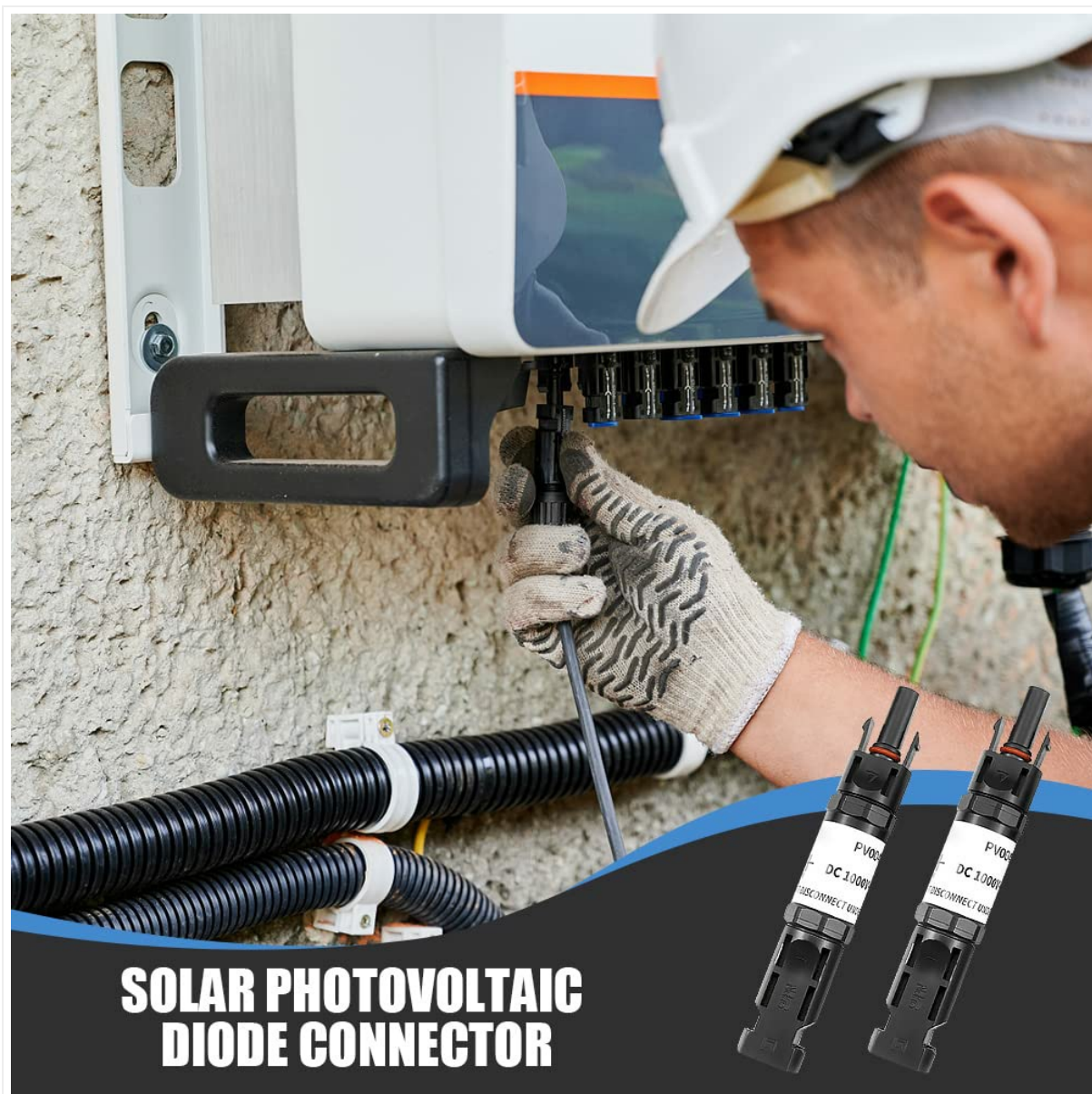
Figure 4.1: Example of connecting the solar photovoltaic diode connector.
