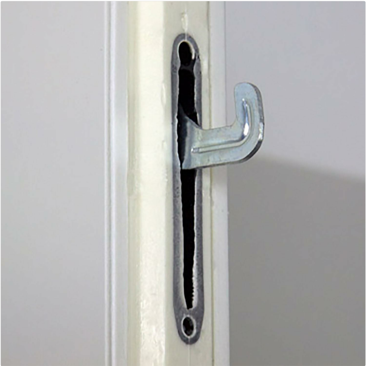
Figure 3.1: Detail of the embedded tensioner for secure panel assembly.
