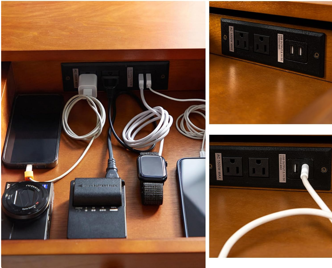
Image: The built-in charging station with AC and USB outlets located within a drawer.
