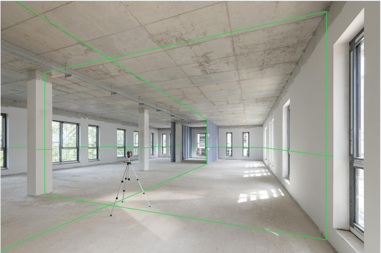
Figure 5.1: The laser level positioned on a tripod in a spacious construction environment, projecting multiple green lines.
