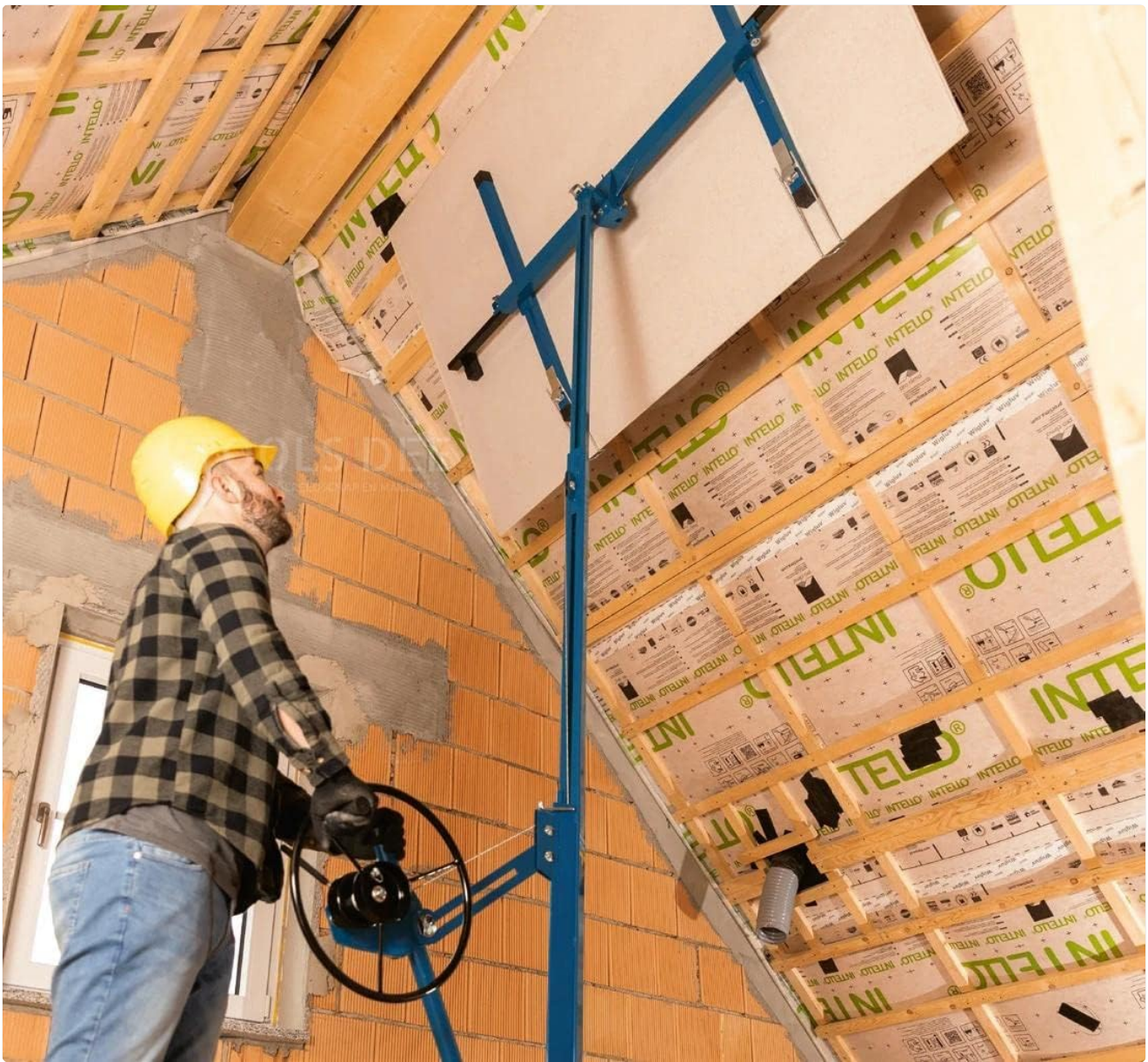
Figure 4: The panel lift with a panel raised to ceiling height and tilted for angled installation.
