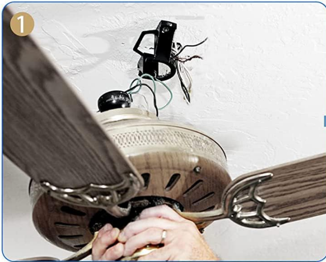
1 Disconnect the ceiling fan wiring
