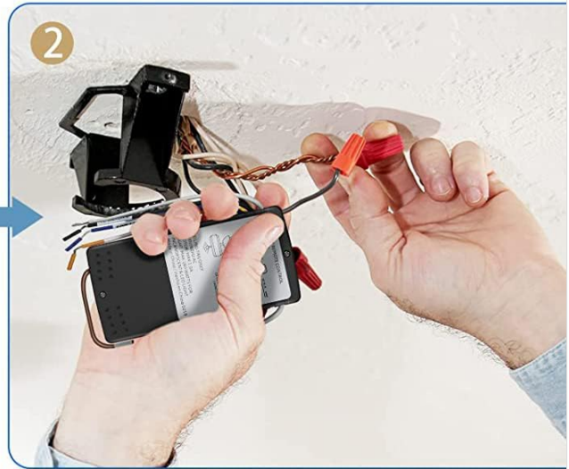
2 Install the controller according to the cable
