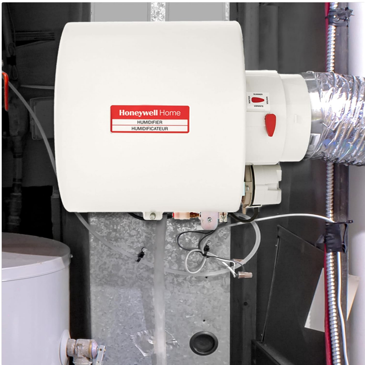
The Honeywell Home HE240D Humidifier unit mounted on the side of a furnace duct, with water and electrical connections visible.
