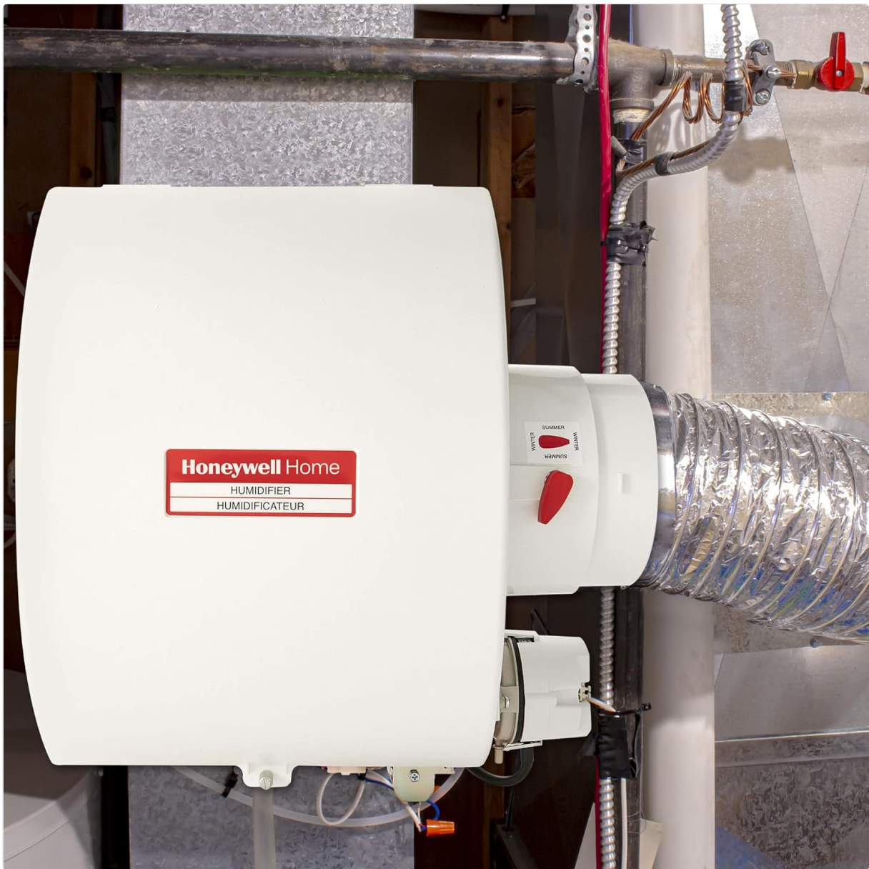
Image: The Honeywell Home HE280D2001/U Humidifier unit shown mounted on the side of a furnace's return air duct, connected to a flexible duct for air circulation.
