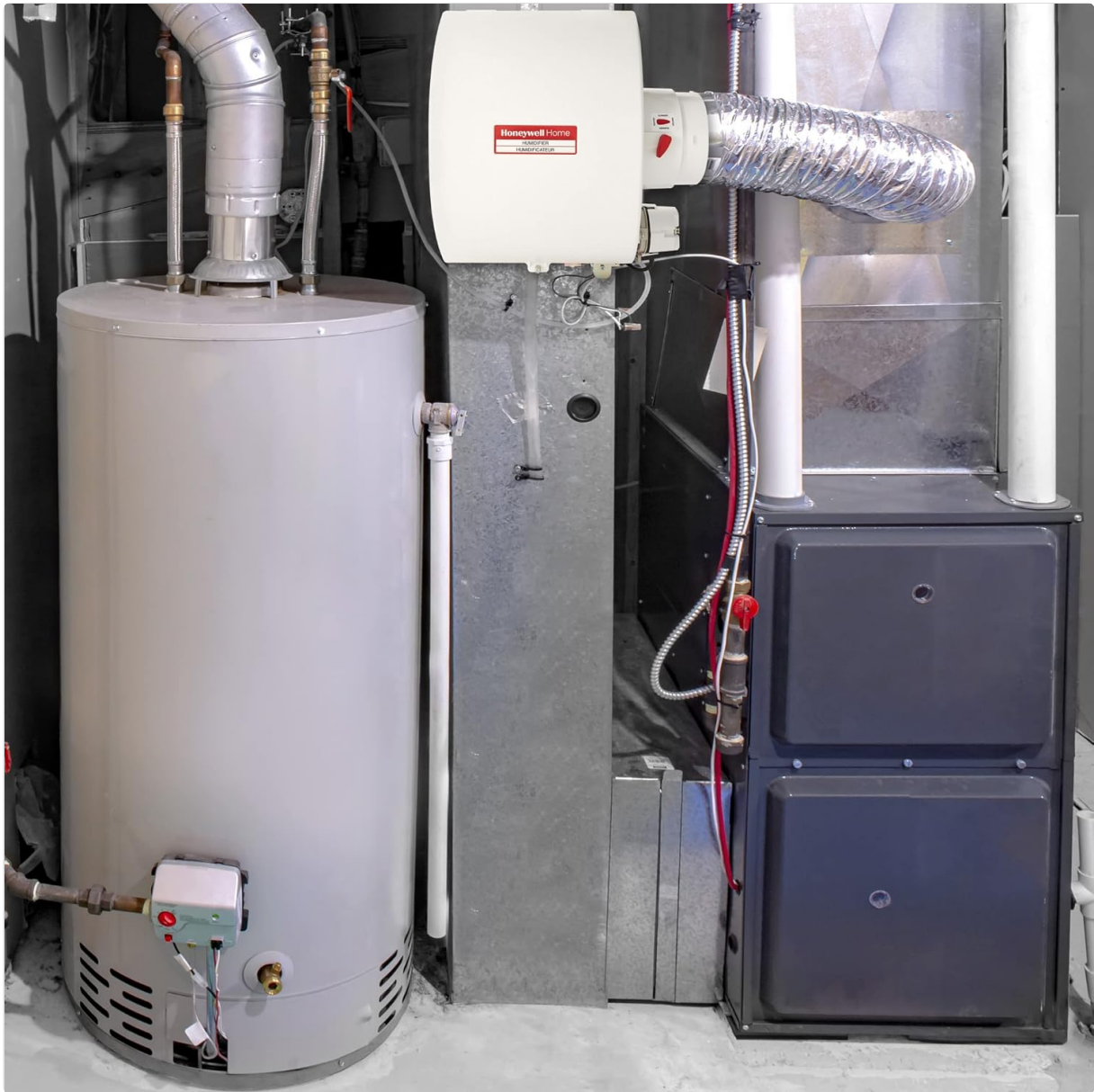
Image: A complete HVAC system installation, showing the Honeywell Home HE280D2001/U Humidifier integrated with a furnace and water heater, demonstrating a typical setup.
