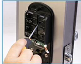
8. Secure the back panel of the door with screws.
