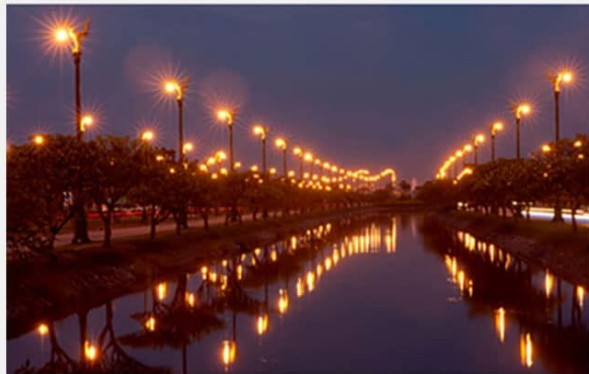
Street Light Control
