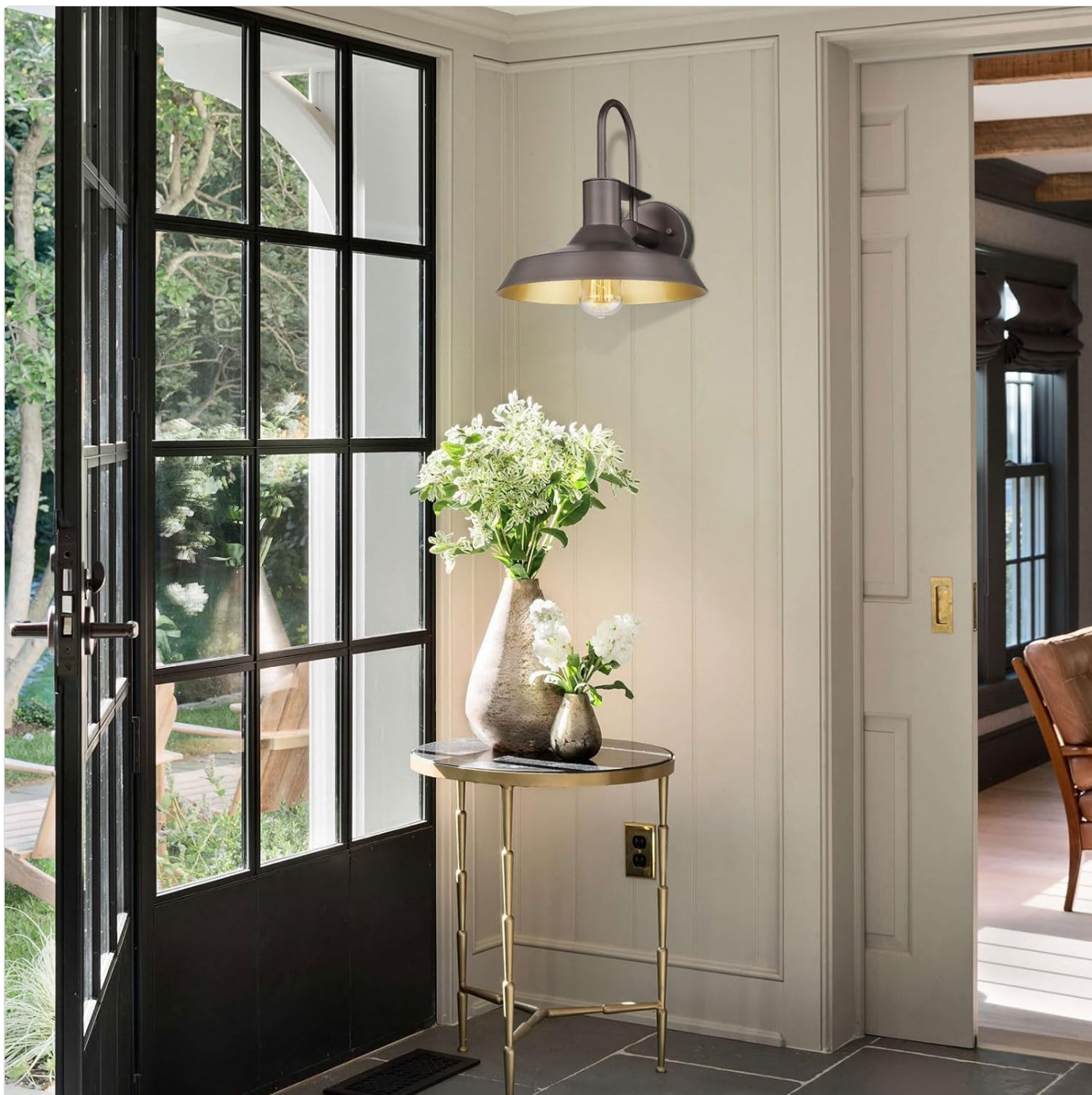
Figure 4: Example of the light fixture installed in an entryway.
