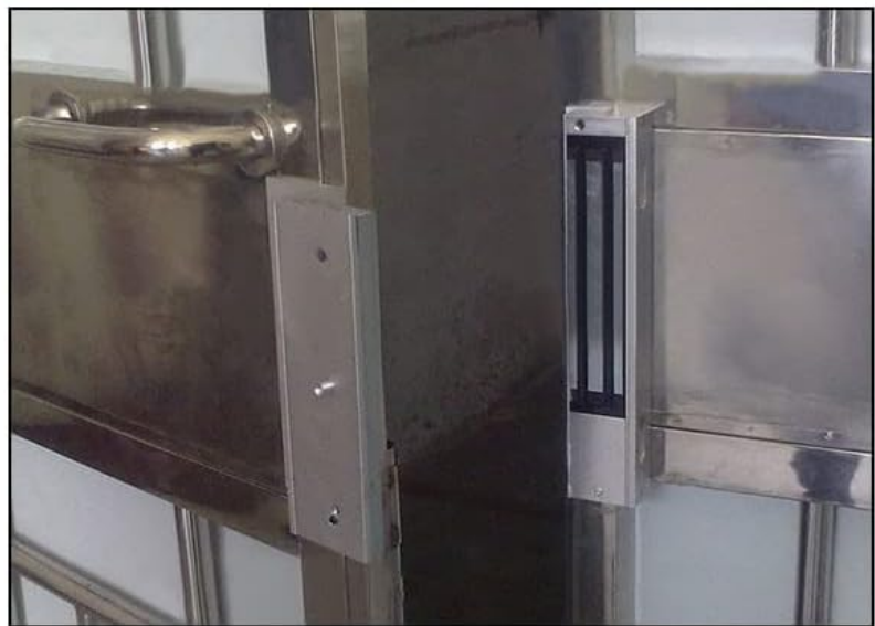
Figure 4: Examples of magnetic lock installation on different door types, including wooden, glass, metal, and fireproof doors.
