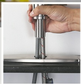
1. Put all hoses into sink hole
