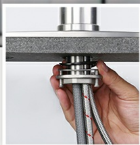
2. Tighten the gasket, washer & U-nut with screws
