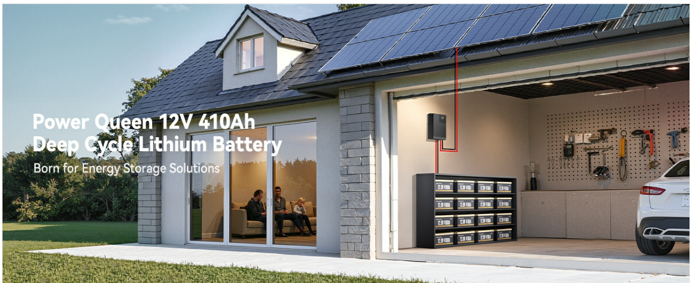
Image: Power Queen 12V 410Ah Deep Cycle Lithium Battery integrated into a home energy storage system.
