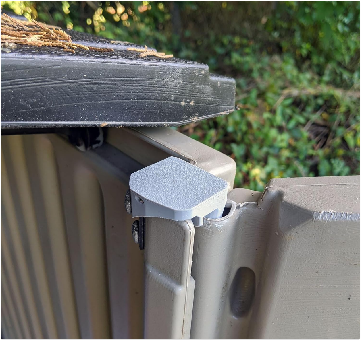
Image: Top view of the hinge during installation, showing alignment.
