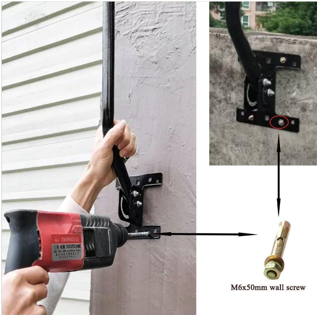
Image 5.2: Wall Mounting Example. This image demonstrates the process of drilling holes and securing the mounting bracket to a wall using wall screws.
