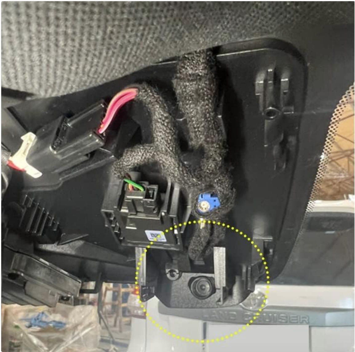
Image 3.4: The dash cam unit securely mounted in its housing, with the lens visible.
