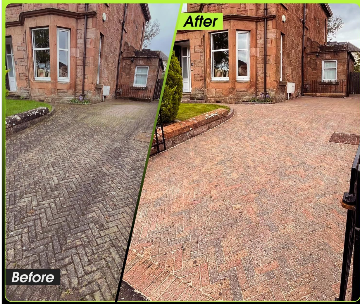
Image: A split image showing a dirty brick driveway 'Before' cleaning and a significantly cleaner driveway 'After' using the pressure washer.
