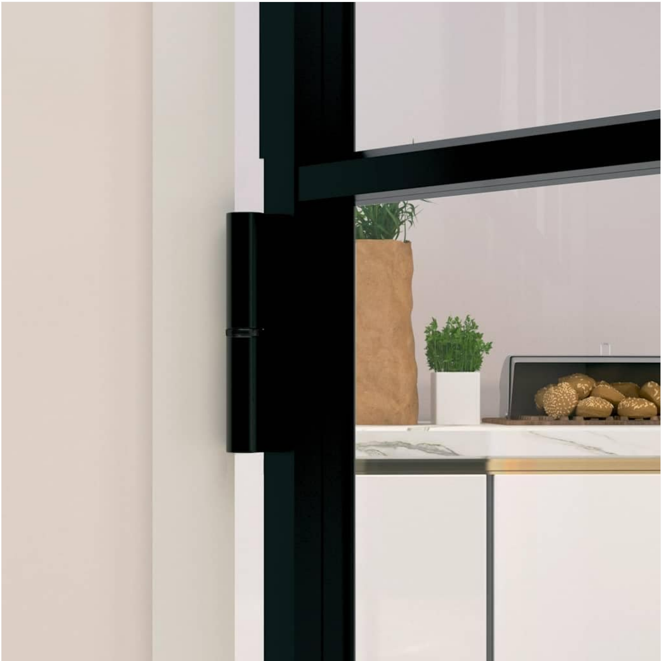
Image 4.3: Detail of the door hinge.
