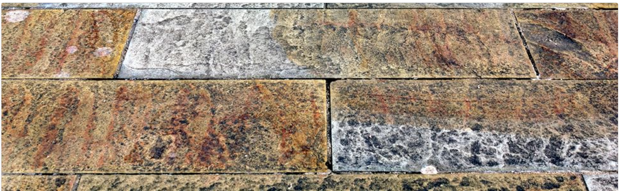
Image 5.4: Before and after treatment of a stamped concrete surface.
