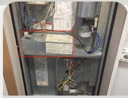
STEP 3 Location the control box.
