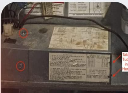
STEP 4 Remove the box cover.
