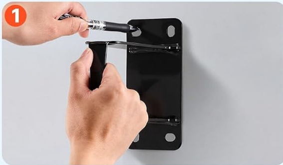
Mark Mounting Position on Wall
