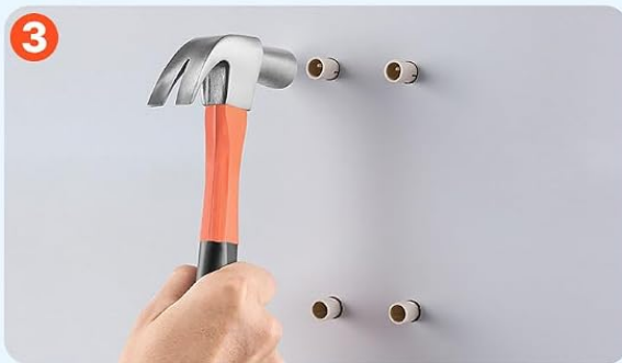
Insert Wall Anchors
