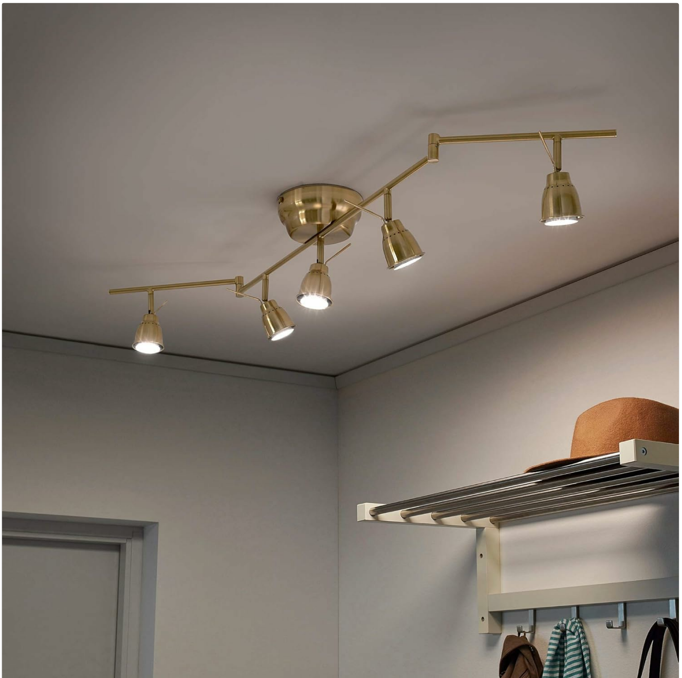
Image 4.1: The Barometer track light installed on a ceiling, demonstrating its placement and illumination.
