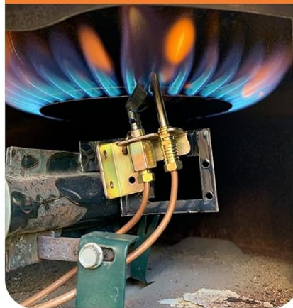
Image 5.1: Visual representation of symptoms indicating a faulty burner receptacle.
