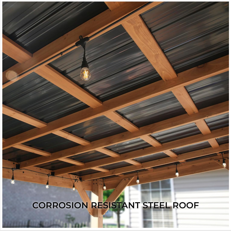
View of the underside of the corrosion-resistant steel roof, showing its robust construction and seamless integration with the cedar frame.
