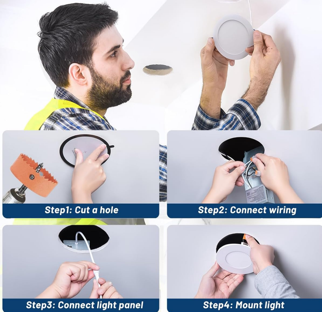
Image 5.1: Visual guide for the installation process, showing steps for cutting the hole, connecting wiring, connecting the light panel, and mounting the light.
