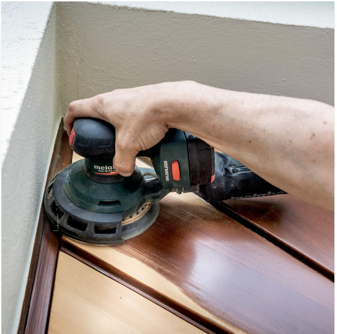
Image 5.3.1: Proper hand placement and technique while sanding a wooden surface.
