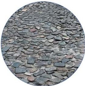
Stone Pavement Road
