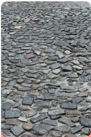
Stone Pavement Road
