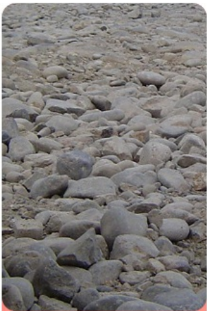
Uneven & Irregular Road
