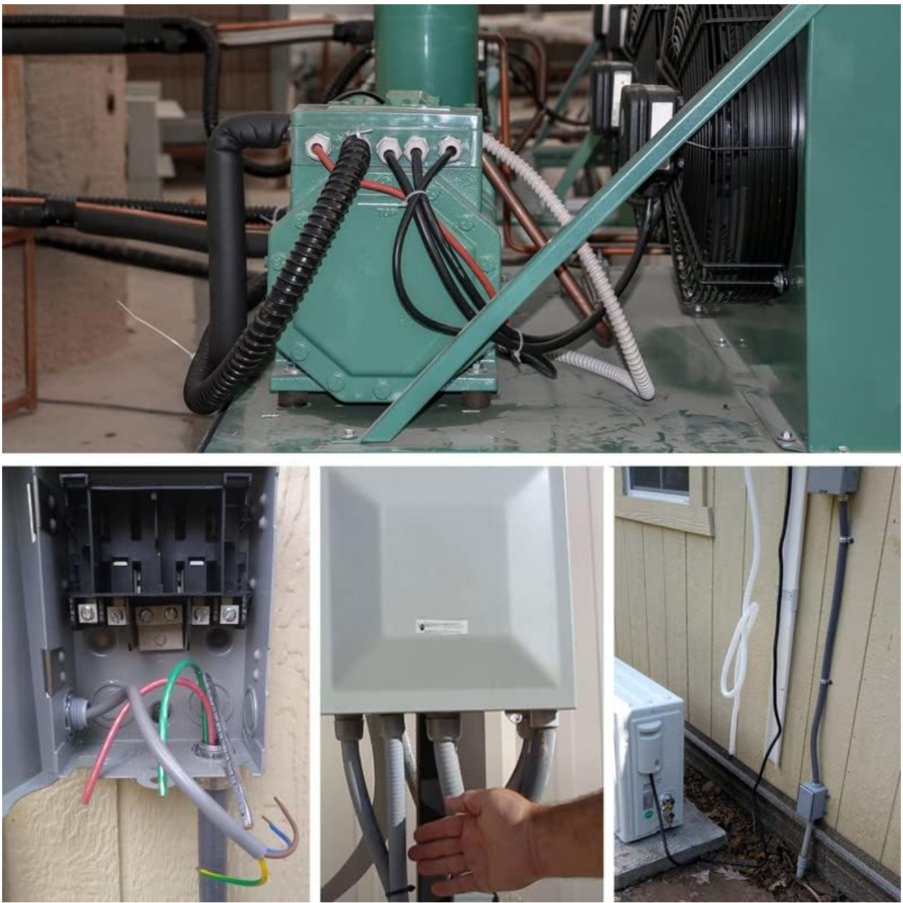
Image 7: A collage of images depicting the liquid-tight conduit installed in various settings, including an electrical box, an outdoor unit, and a compressor, showcasing its versatility.
