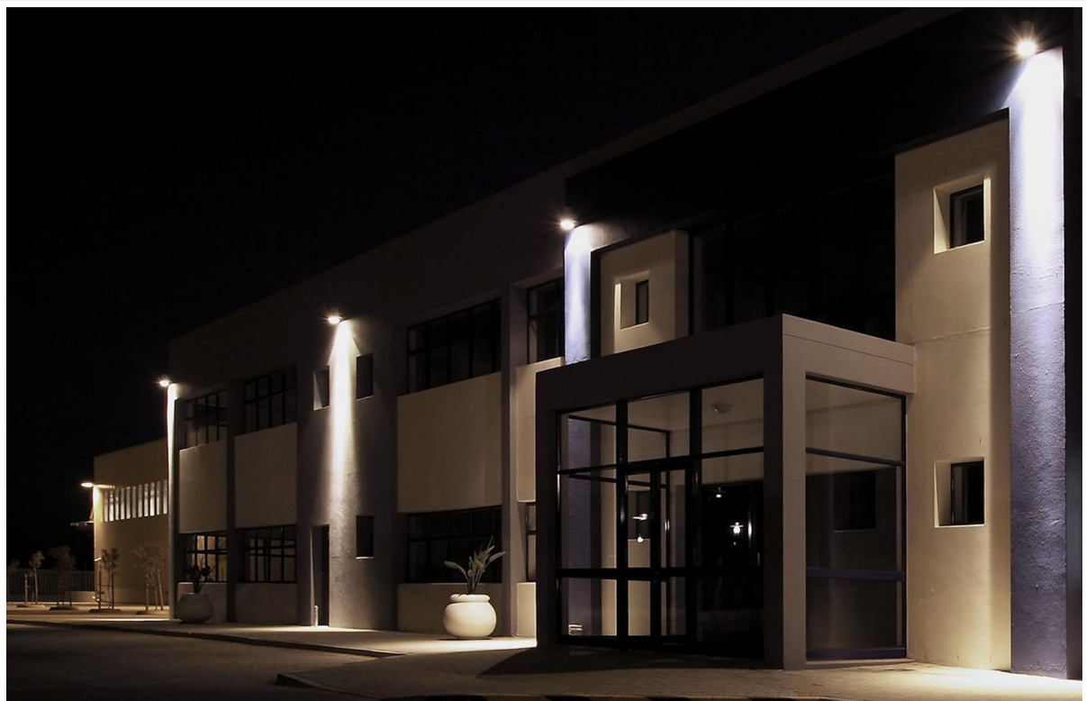
Figure 2: Example of Philips Projectline LED Floodlights installed on a building exterior, providing warm white illumination at night.
