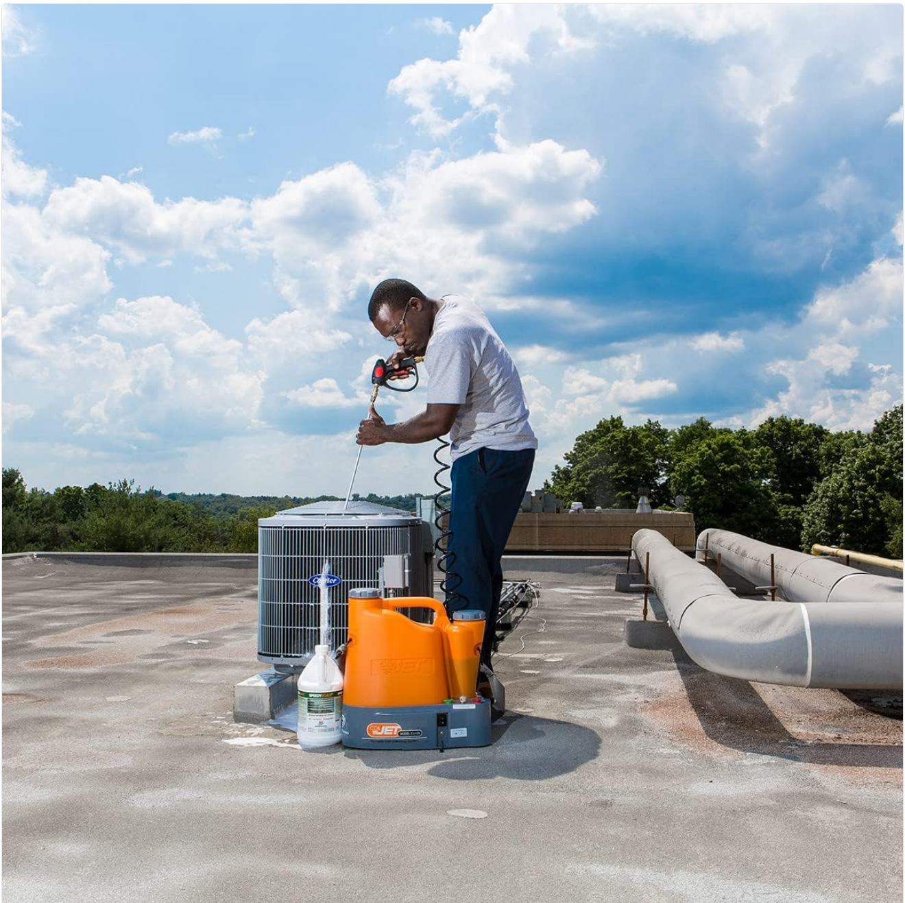
Figure 5: Cleaning a rooftop HVAC unit.
