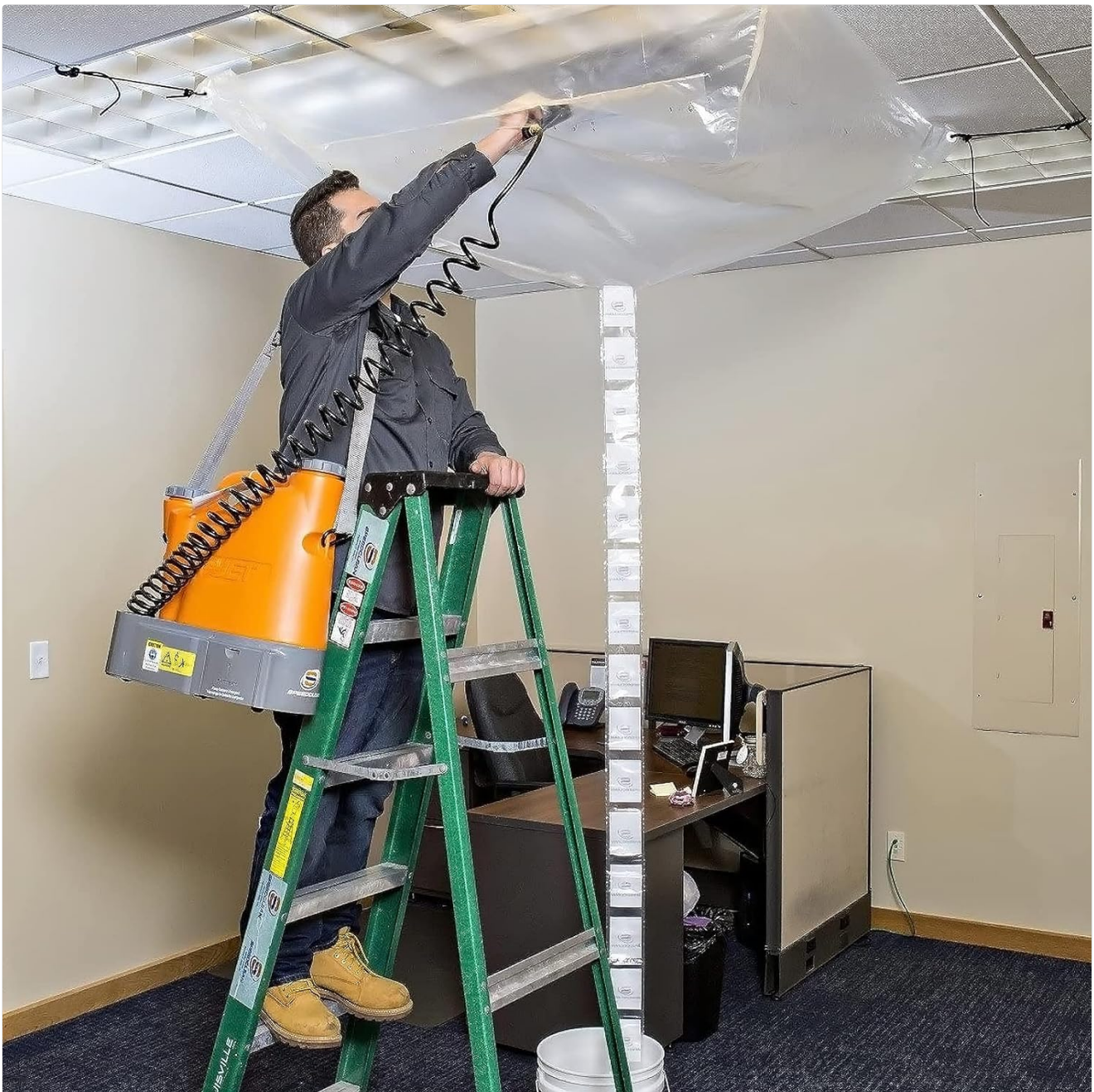
Figure 4: Cleaning an indoor evaporator unit from a ladder.
