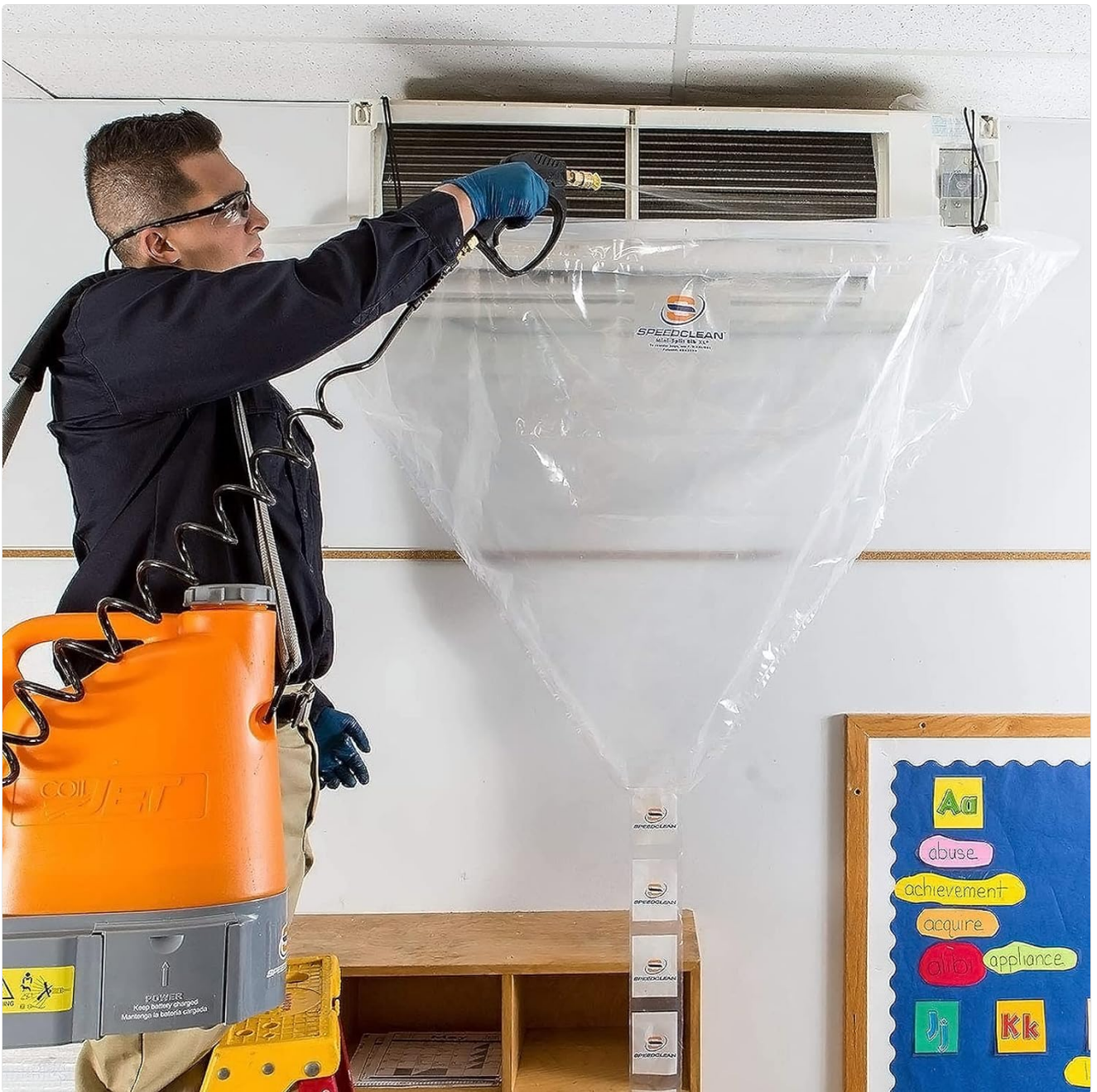
Figure 3: Cleaning an indoor evaporator unit using a containment bib.
