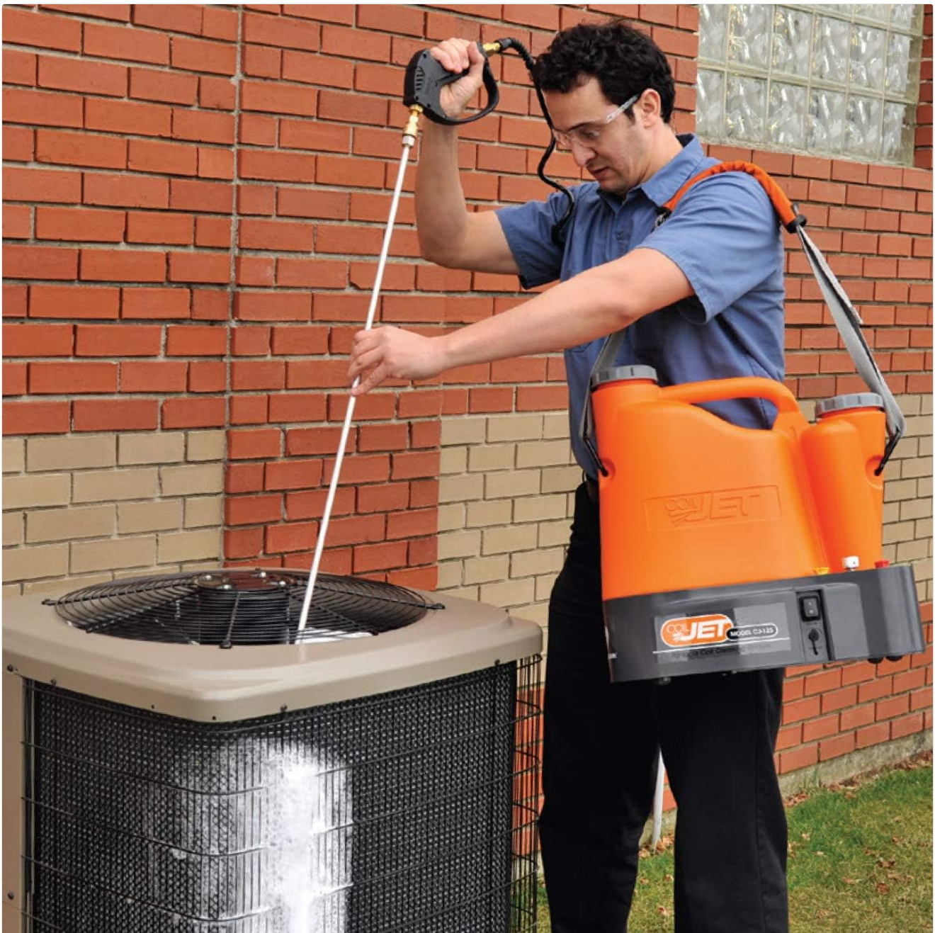
Figure 2: Cleaning an outdoor condenser unit.
