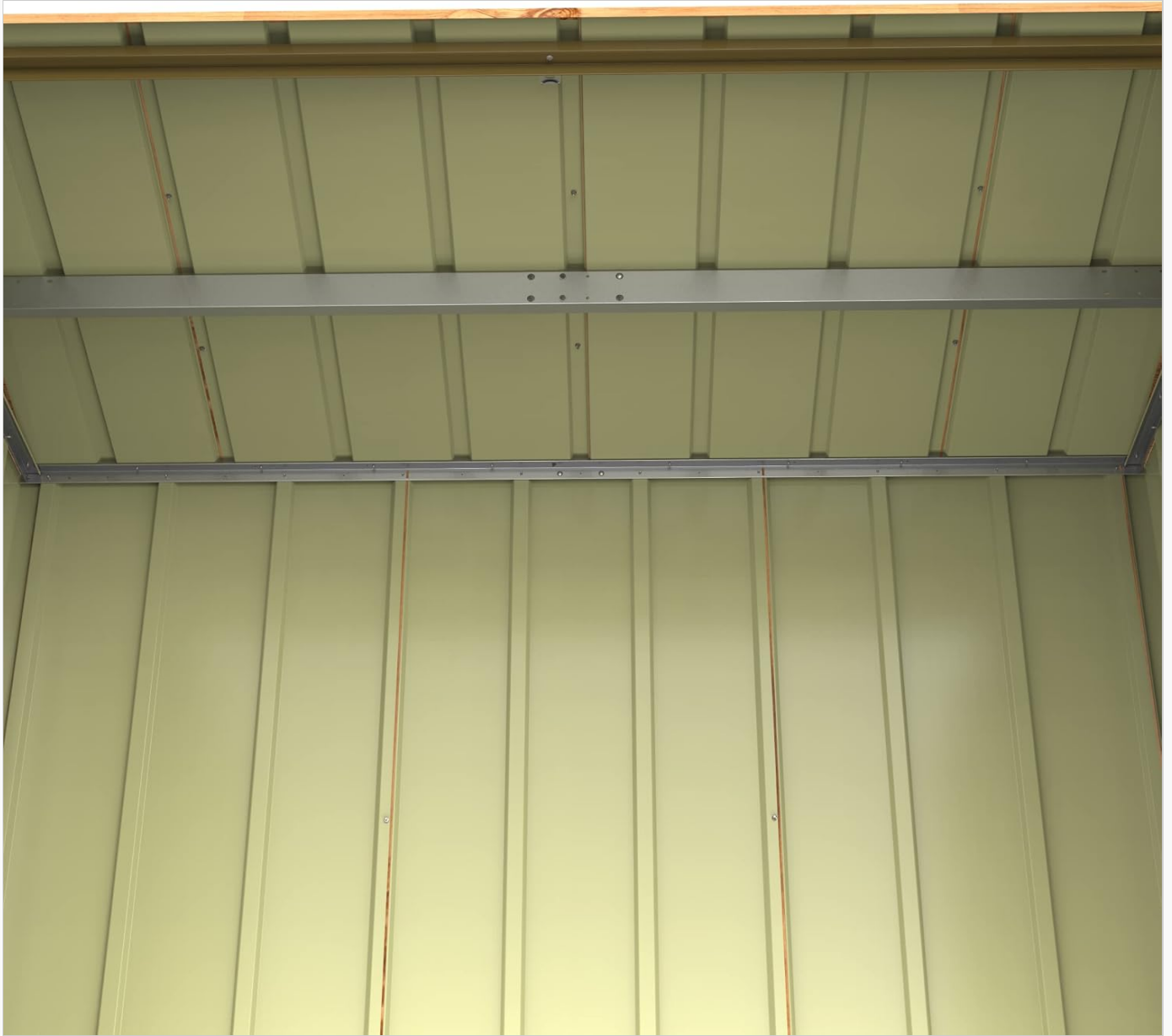
Figure 2.8: Interior view showing the robust metal roof structure and internal framing.
