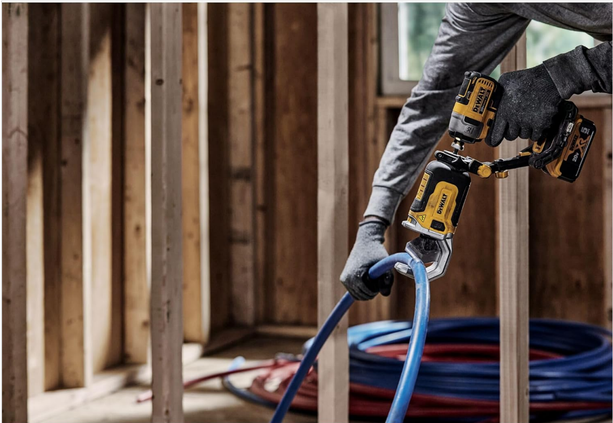
Figure 5: The cutter is also effective for cutting PEX piping.
