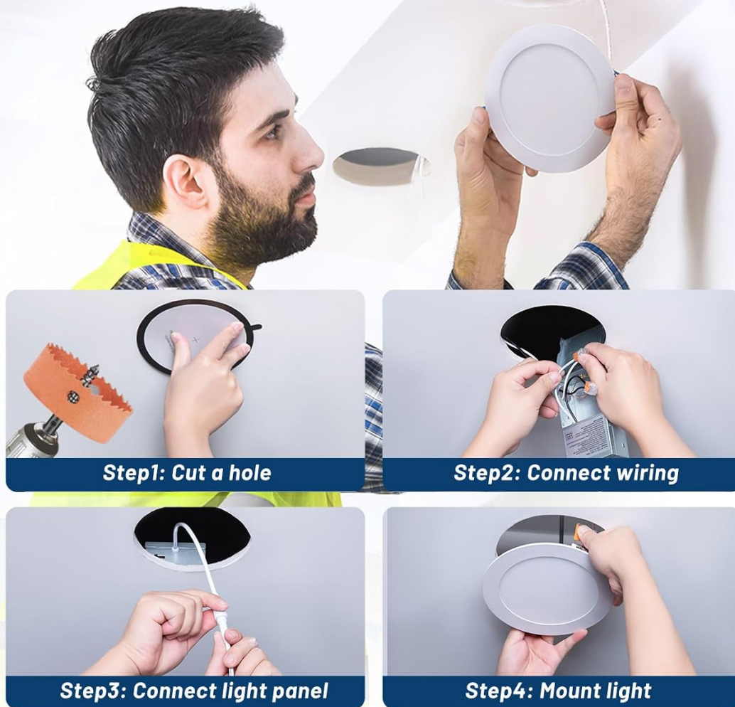
Image 3: A four-step visual guide demonstrating the easy installation process: 1. Cut a hole, 2. Connect wiring, 3. Connect light panel, 4. Mount light.
