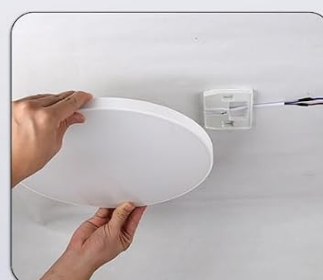
4. Secure the lamp body to the base
