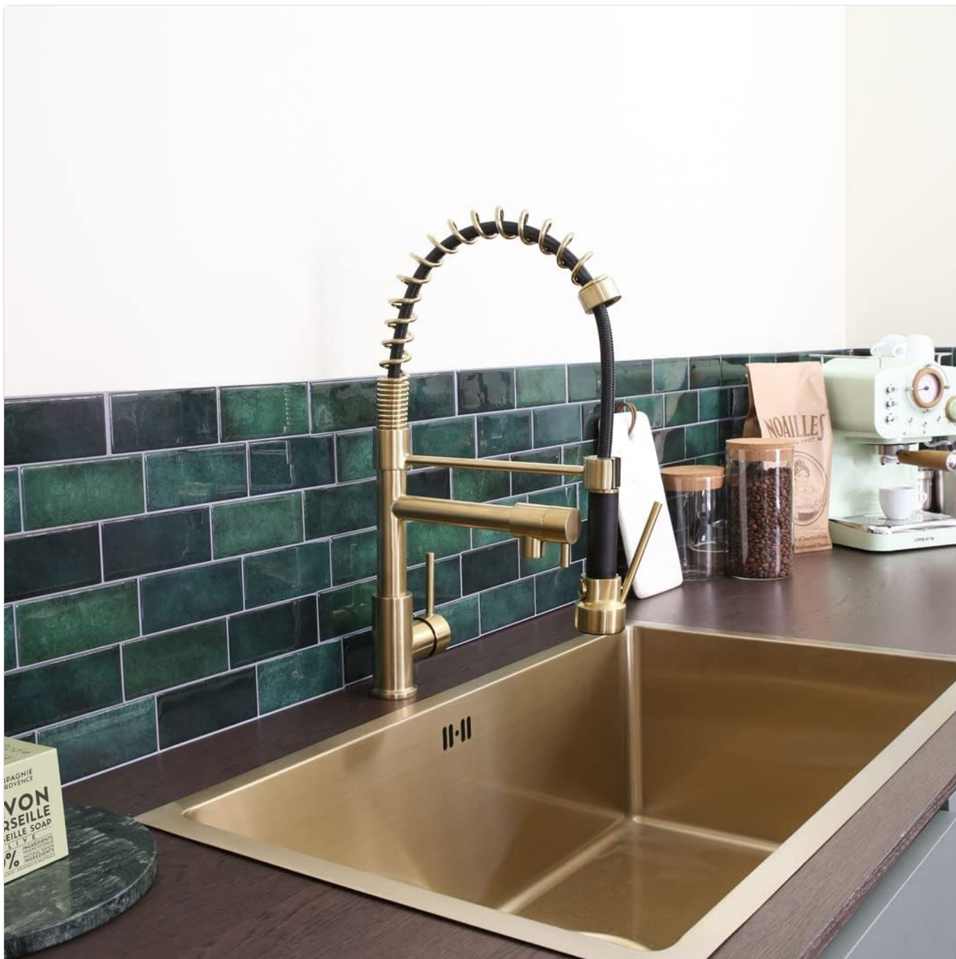
Image: The ESSEBAGNO Big Pro 9019781 kitchen faucet, featuring a gold finish and a mobile spray head, installed in a kitchen setting.
